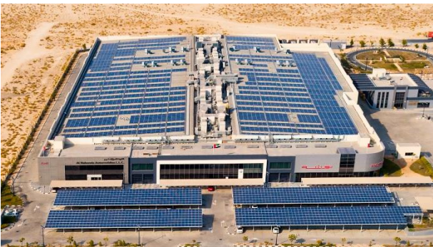
The solar plant at Al Nabooda Automobiles, Body & Paint Shop and Test Facility in Dubai Industrial City
